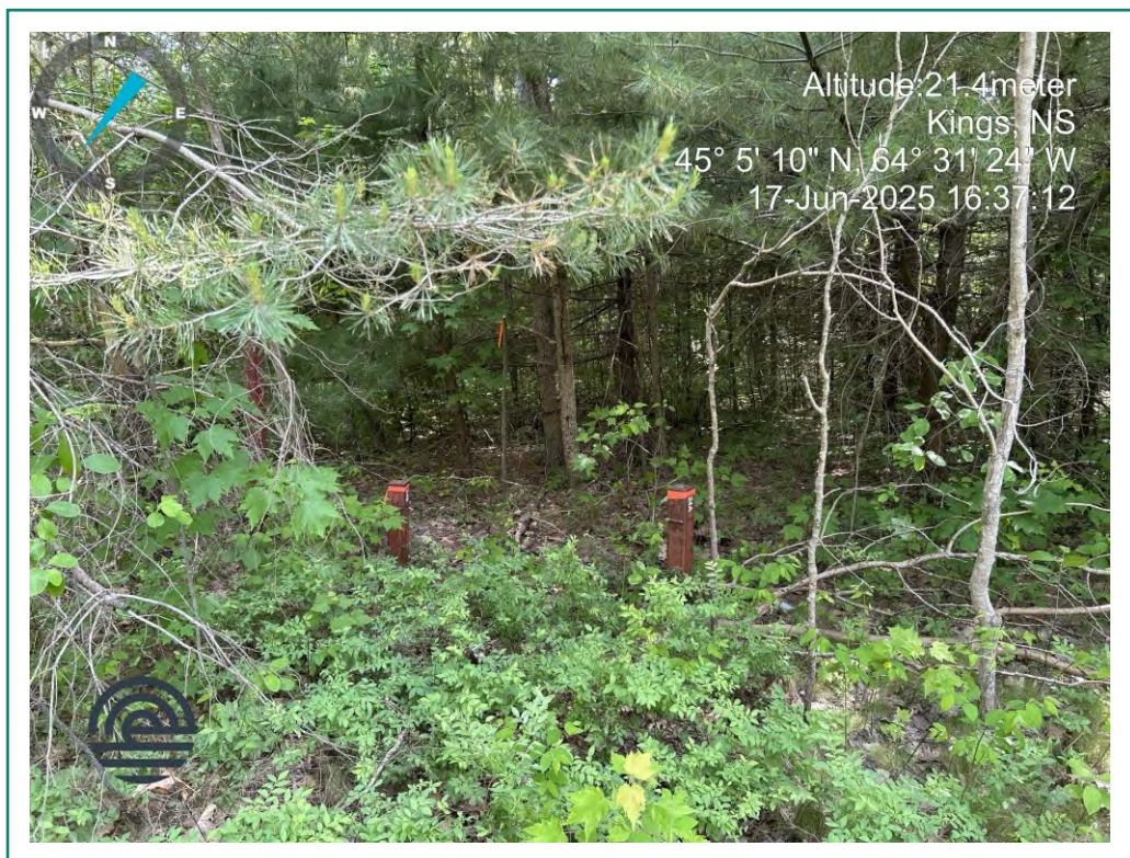
Photo 20: Monitoring Wells MW24 A (right) and MW24B (left).
